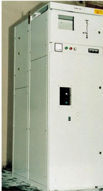
Figura 27 Tablero de conexiones o Switchboard . Tomada de ( ESP Expert , s/f).
