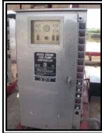
FIGURA 32. Bomba Diesel Contraincendios
